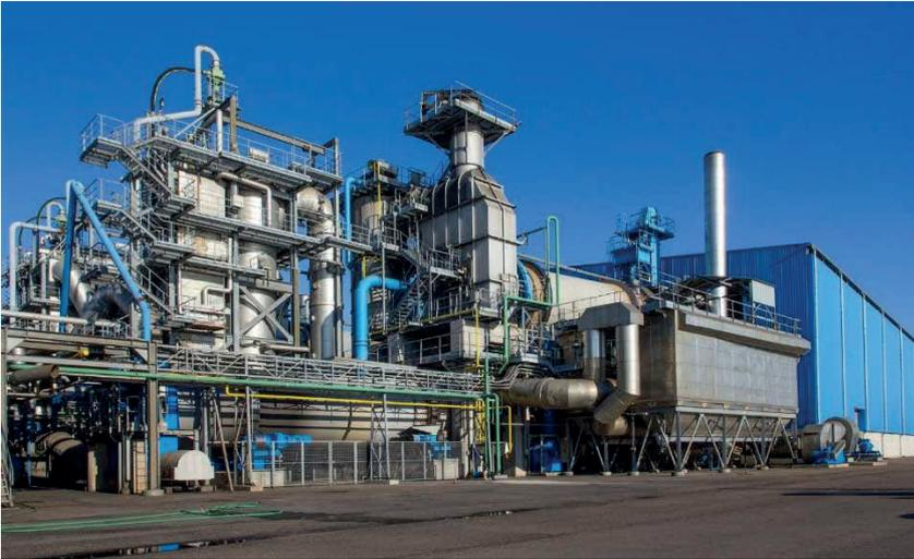
*Complete flue gas cleaning system downstream from a special waste incineration plant with waste heat boiler and steam turbine*
